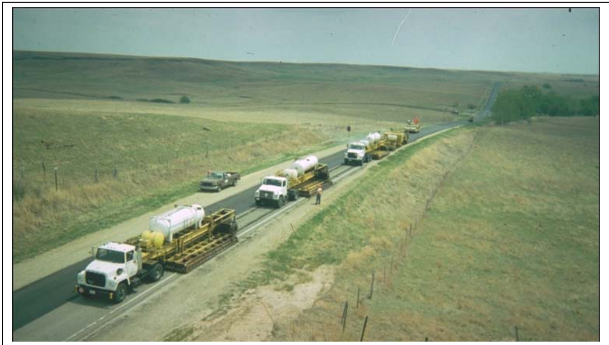
Figure 11. Heater Scarification of HMA Surfaced Pavements
