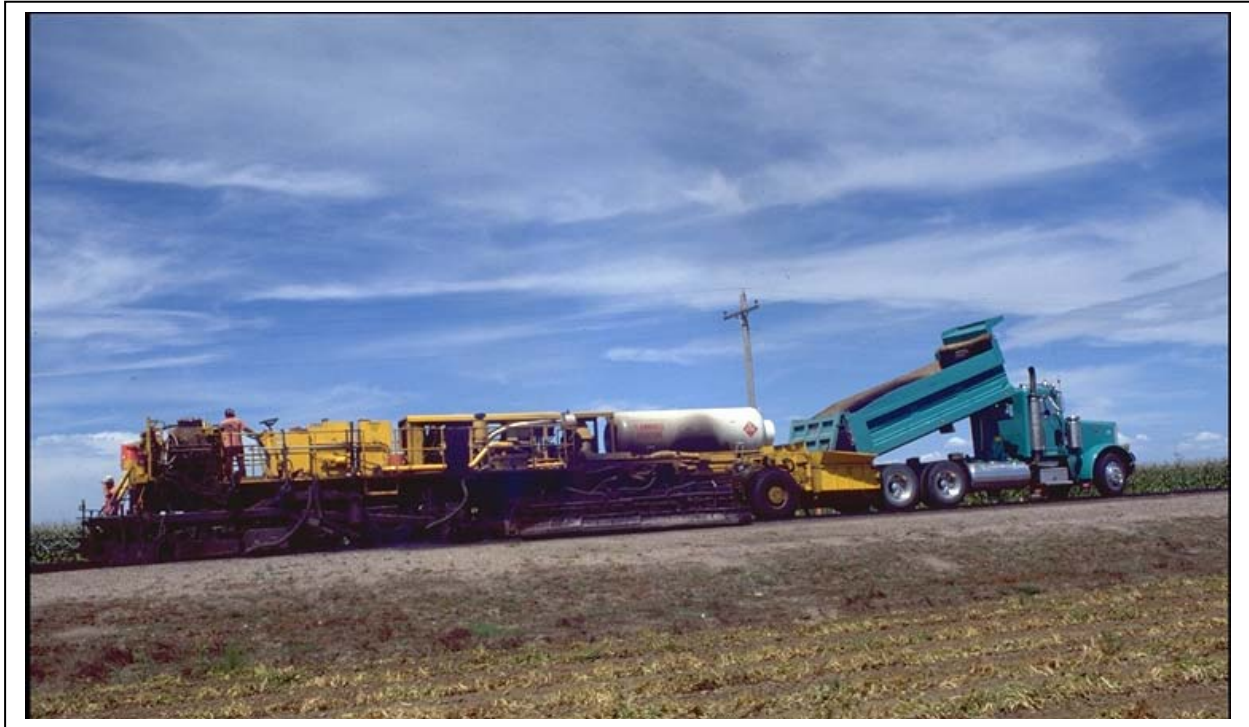
Figure 10. Hot In Place Recycling Method of Flexible Pavement
