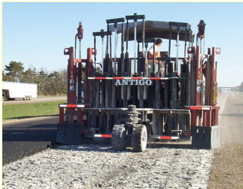
Figure 9. Multiple-Drop Hammer for Rubblizing PCC Slabs
