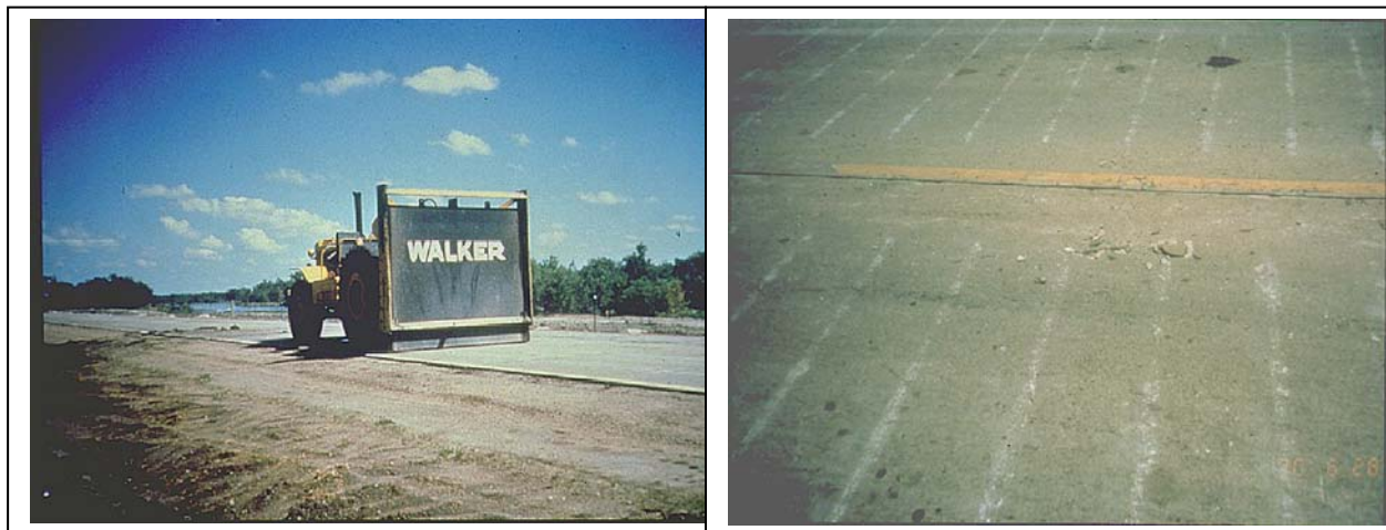
Figure 7. Crack and Seat or Break and Seat Equipment for Fracturing PCC Slabs
