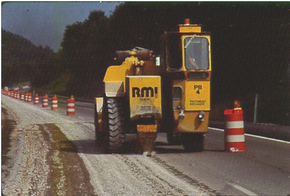
Figure 8. Resonant Frequency Pavement Breaker for Rubblizing PCC Slabs
