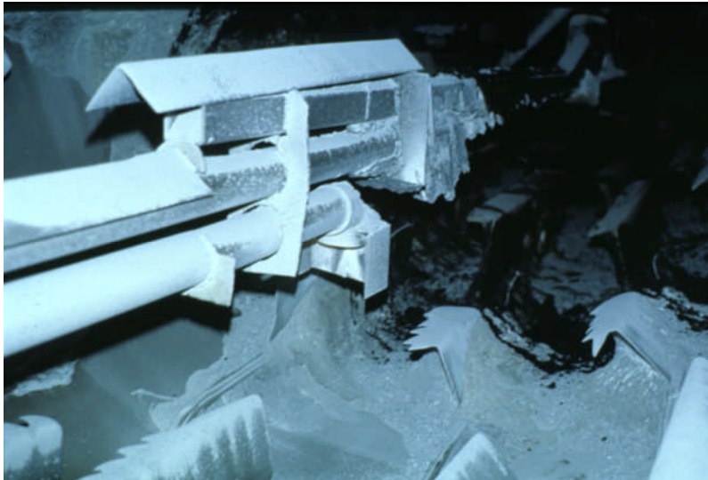
Figure 7: Fiber Injection Point in a Drier-Drum Plant
