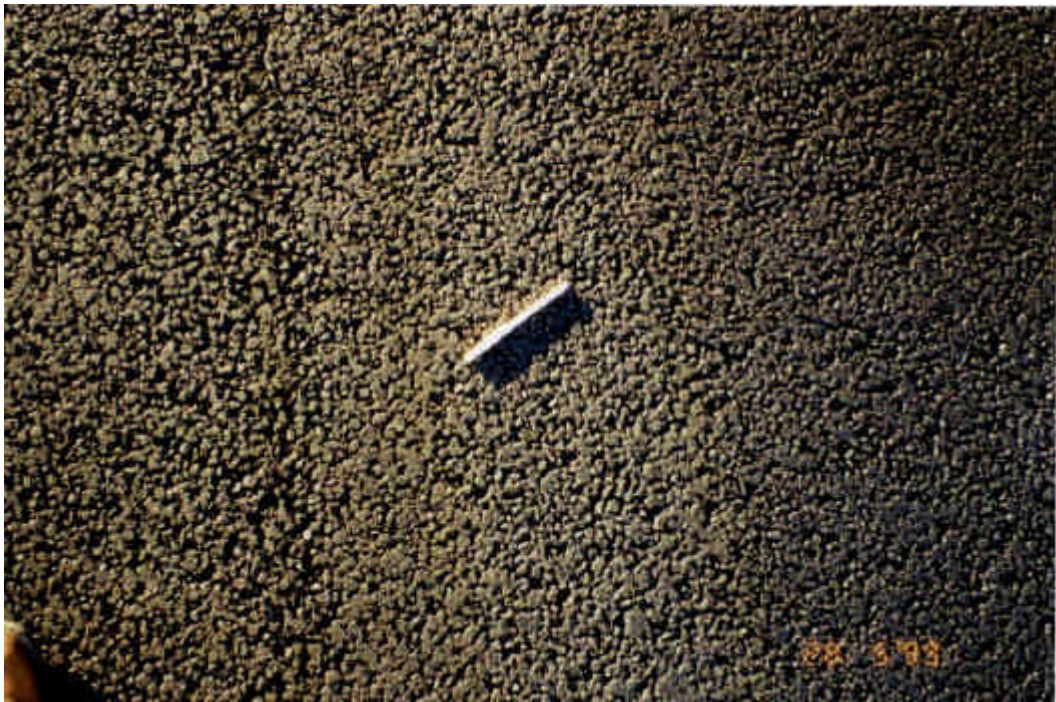
Photo 5 Typical joint between paving lanes
