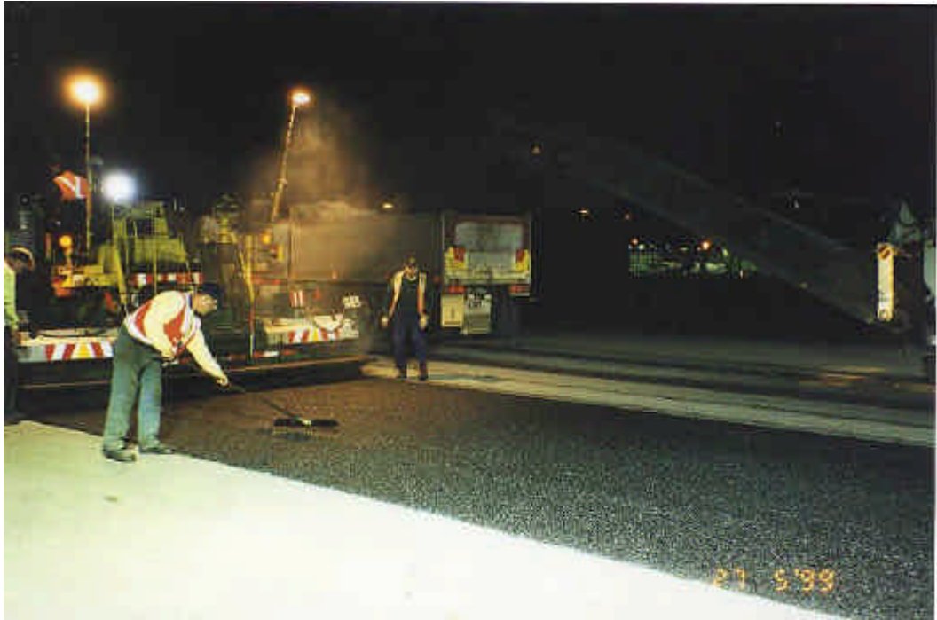
Photo 1 Laying of stone mastic asphalt trial
