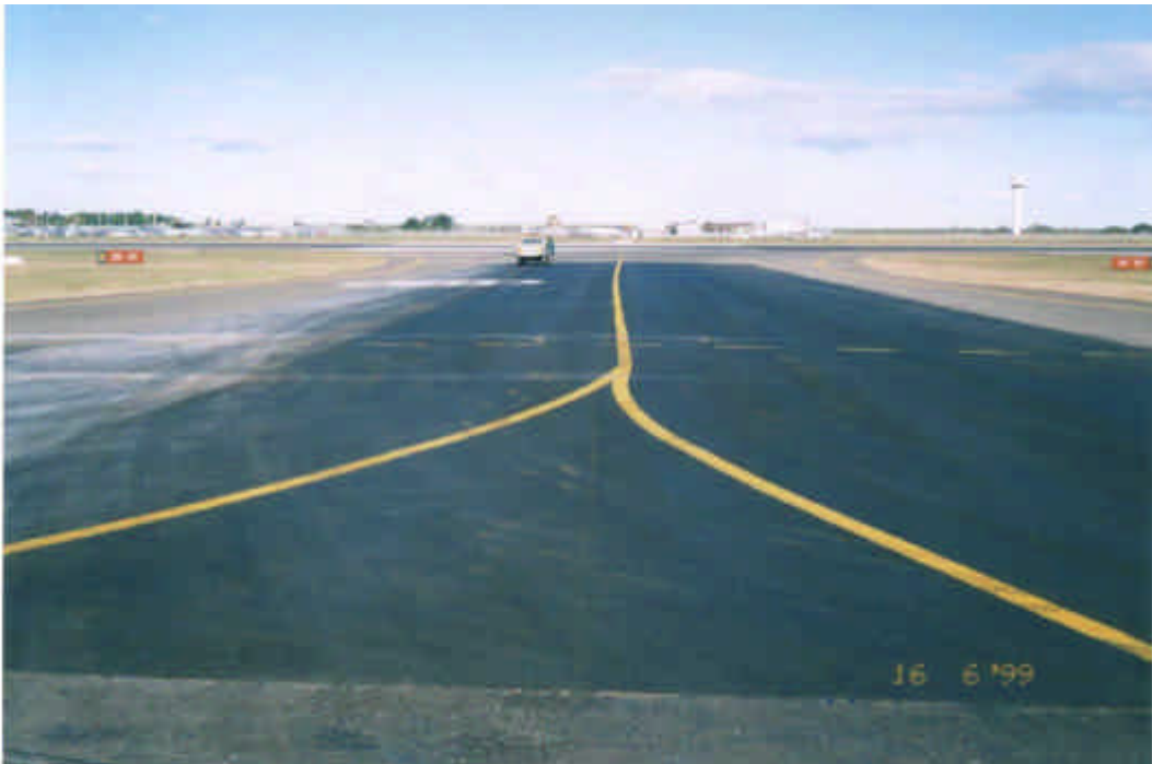
Photo 10 Overall view of trial area looking south
