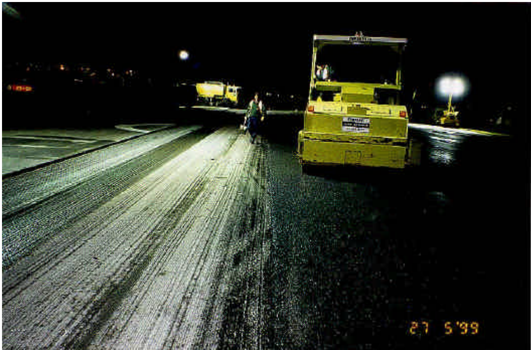
Photo 2 Compaction of stone mastic asphalt trial
