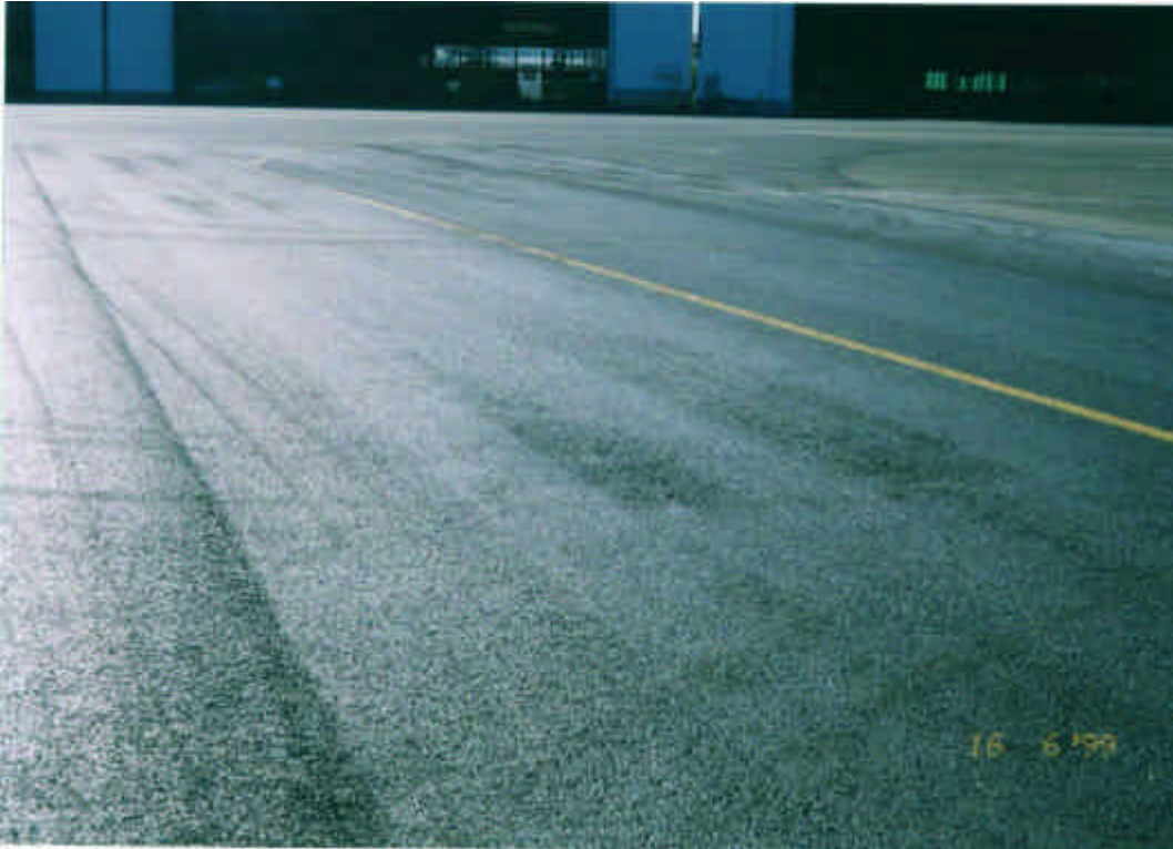
Photo 7 View of trial looking north – note open textured areas
